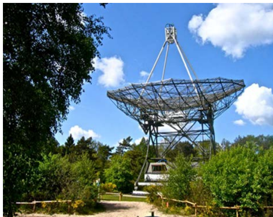
Fig. 3: The Dwingeloo radio telescope in The Netherlands. Inaugurated in 1956, the dish measures 25 metres diameter (courtesy of CAMRAS)
